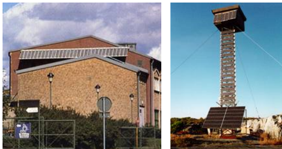
Figure 1: To the left: Sweden's first PV demonstration project in Årsta, Stockholm. To the right: The stand-alone PV system on Bullerö, based on the modules from Årsta.
